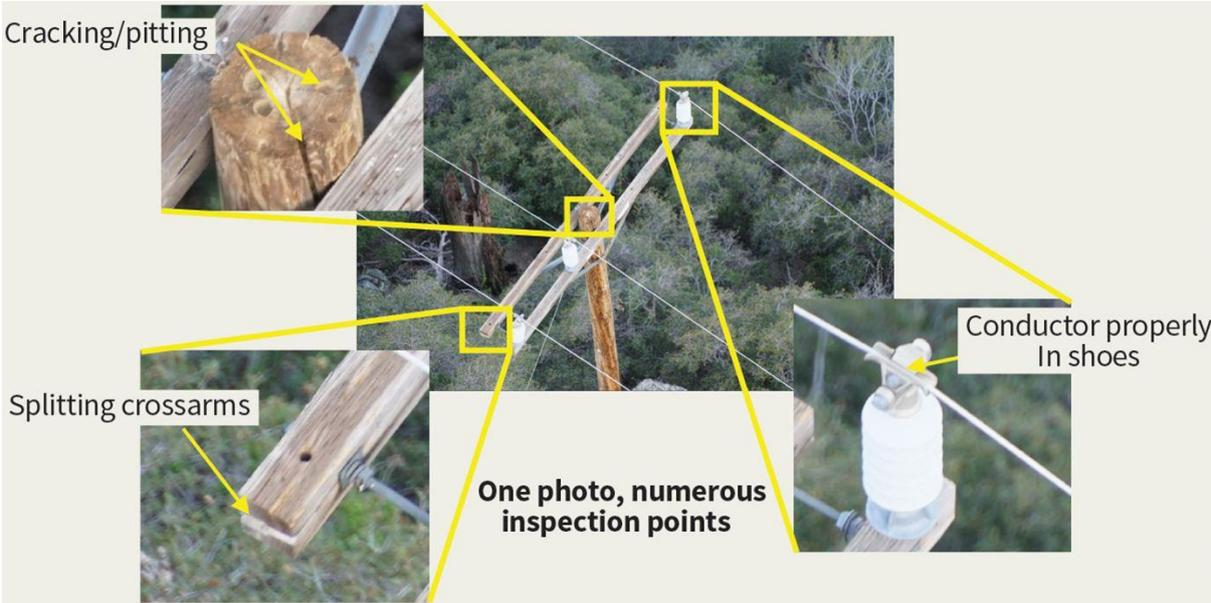
**Fig. 1.14: Inspection points in a photo taken by a drone camera [31]**
