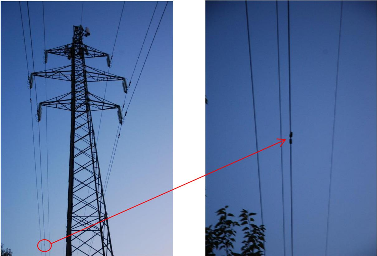
**Fig. 1.5: Slipped vibration dumper mounted on an overhead line**
