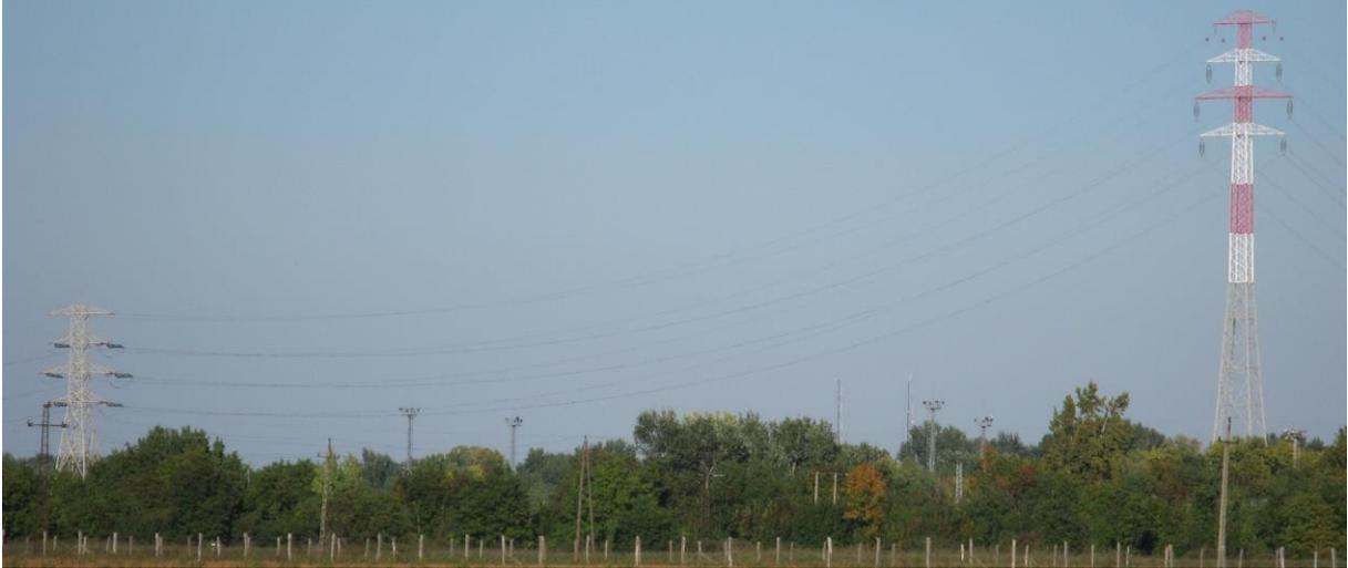
**Figure 3.2: Inclined span in a flat terrain**
