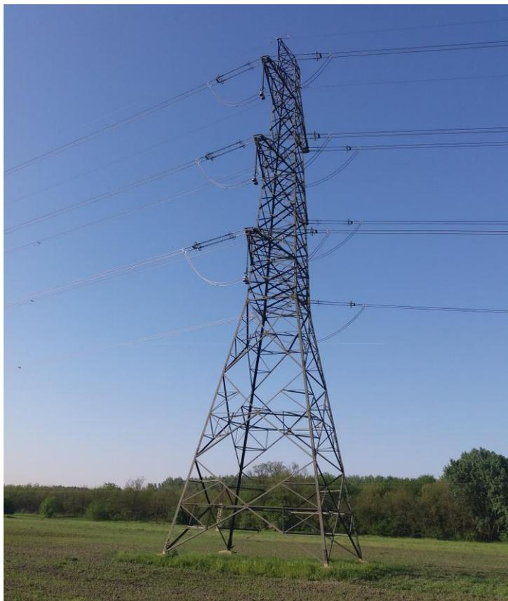
**Fig. 5: The angle tower of transmission line**
