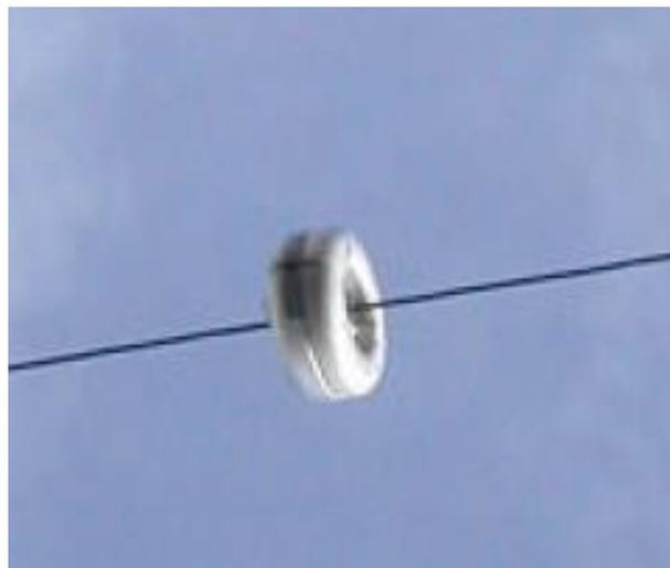
**Fig. 1.9: Conductor temperature sensor attached to the energized conductor [22]**
